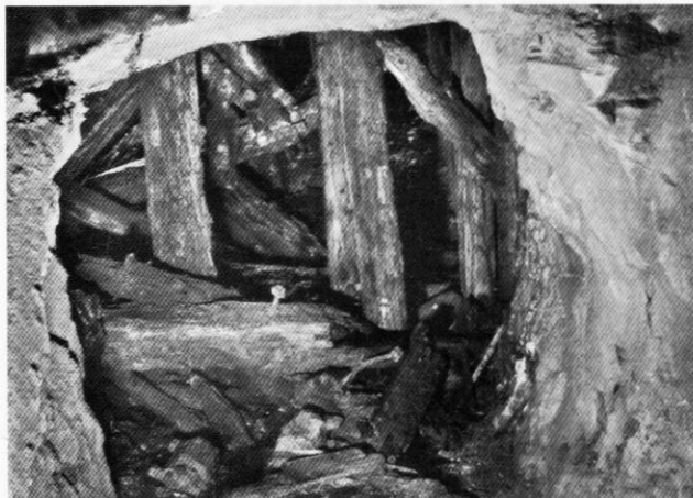
Passage in the 19-Lachter Stollen (1 Lachter = ~1.9 metres)
